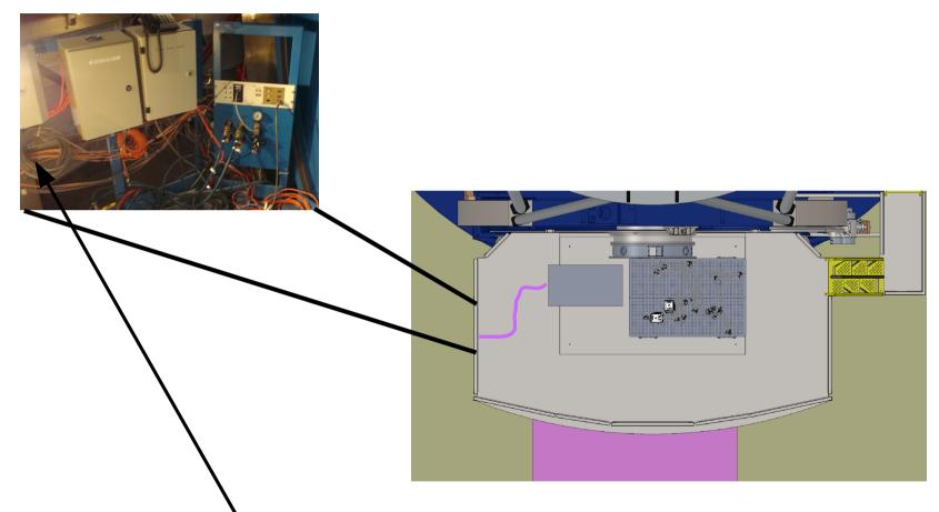
Fiber junction box with 4x pairs 10Gb/s fiber routed to equipment room.
