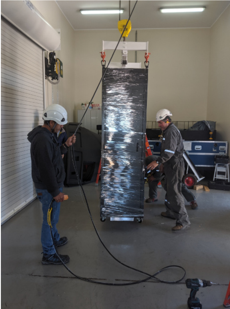
The electronics box rack being lifted.
