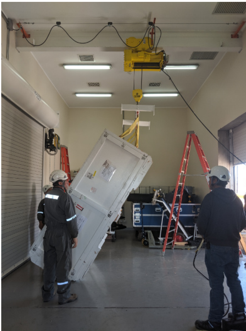
The electronic box being lifted into loading position
