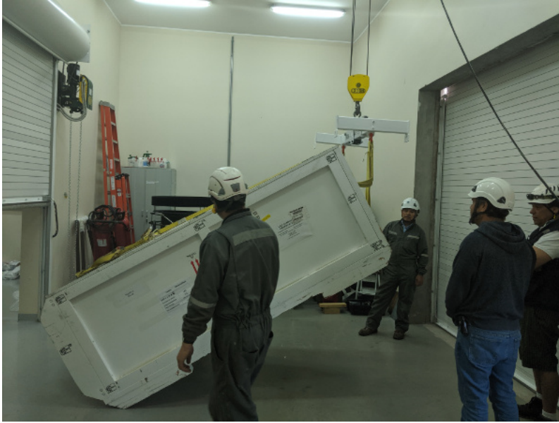
Lowering the electronics box.
