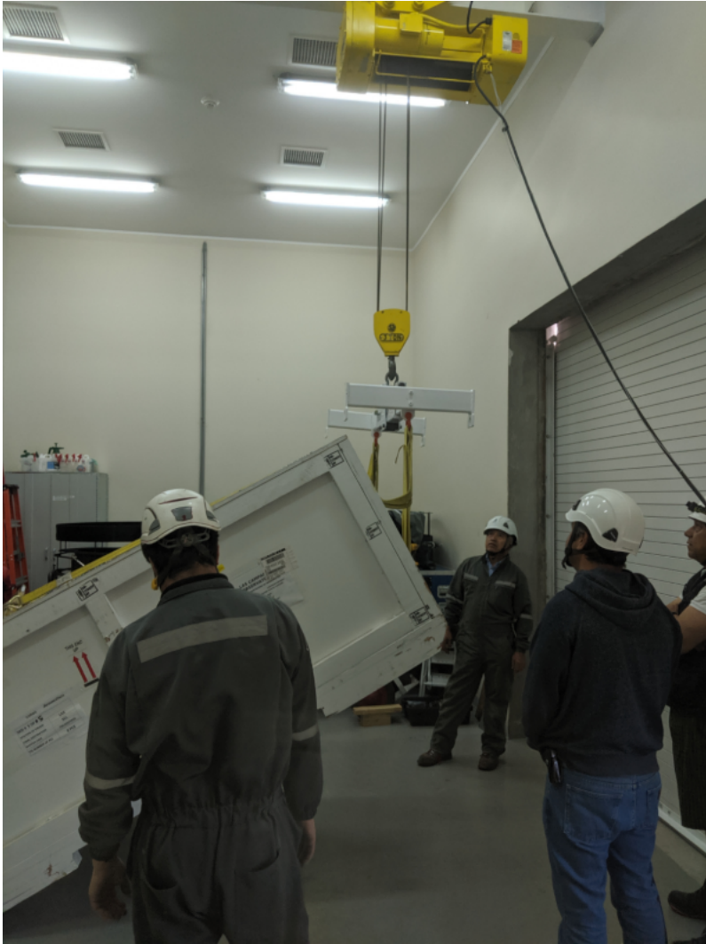
The electronics box being lifted. Note that as it is lifted the crane truck moves to the left.
