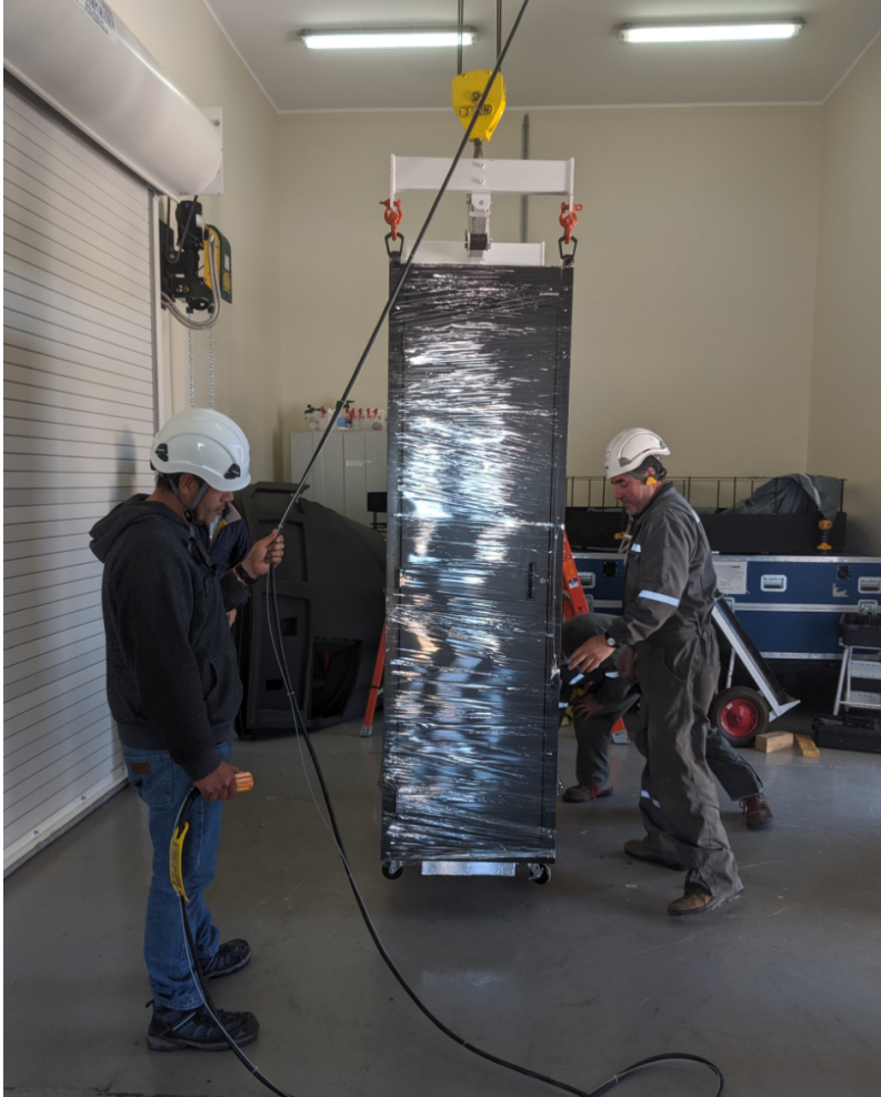
Setting the Rack down.
