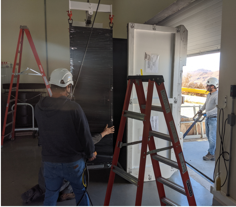
The rack being removed from the box.
