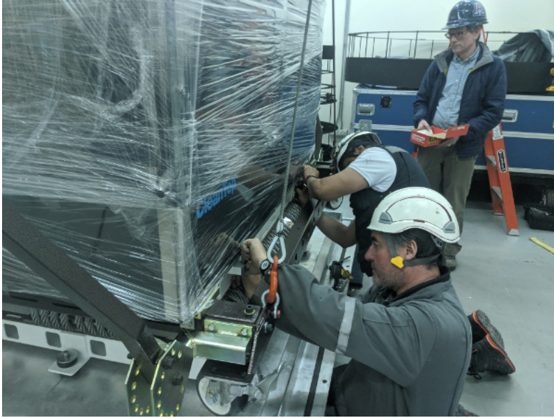
Tightening the bolts.
