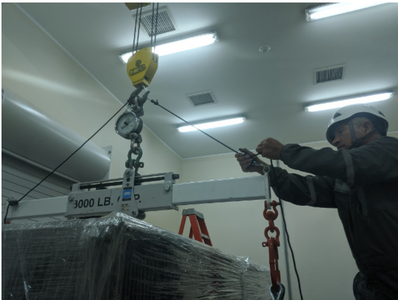
The triangle stabilizing ropes should be tight, but not become the lifting point for the load.
