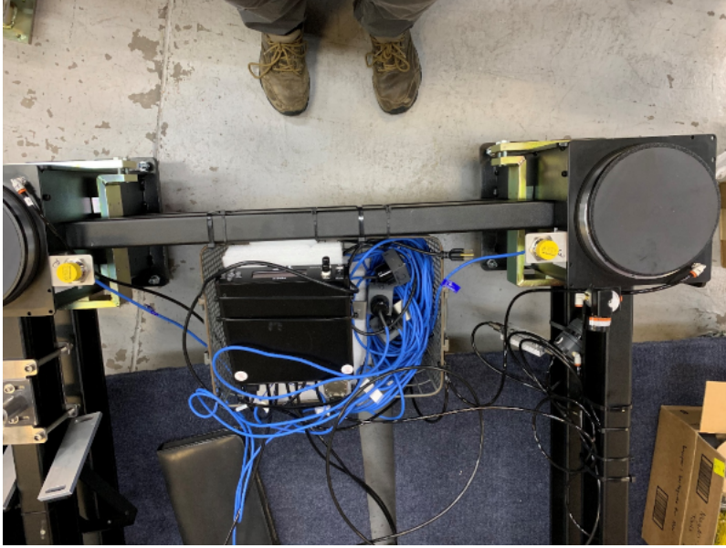
Legs on 2 dollies placed in the middle of the table under each lower long tie bar (away from basket).
