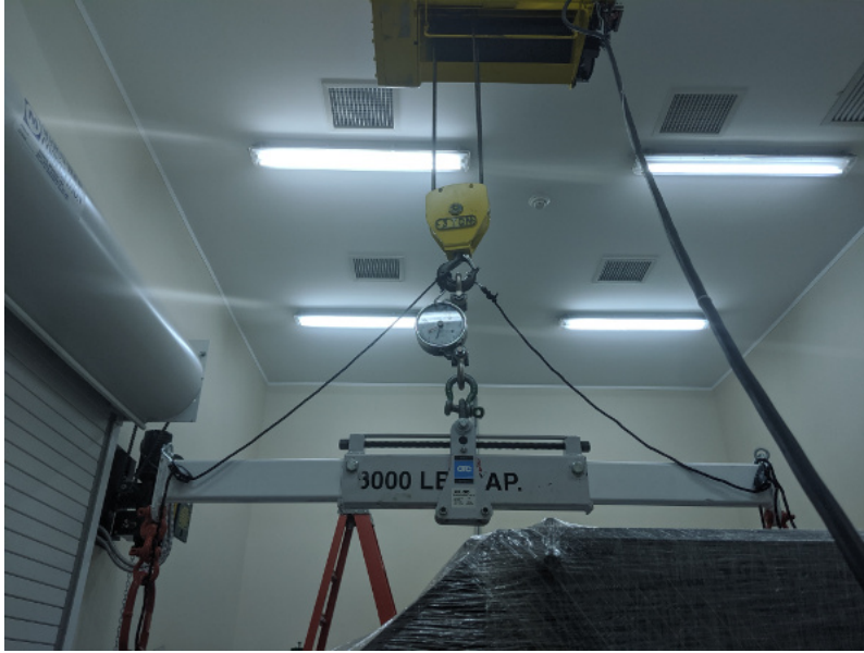
The load spreader attached to the crane for lifting the cart
