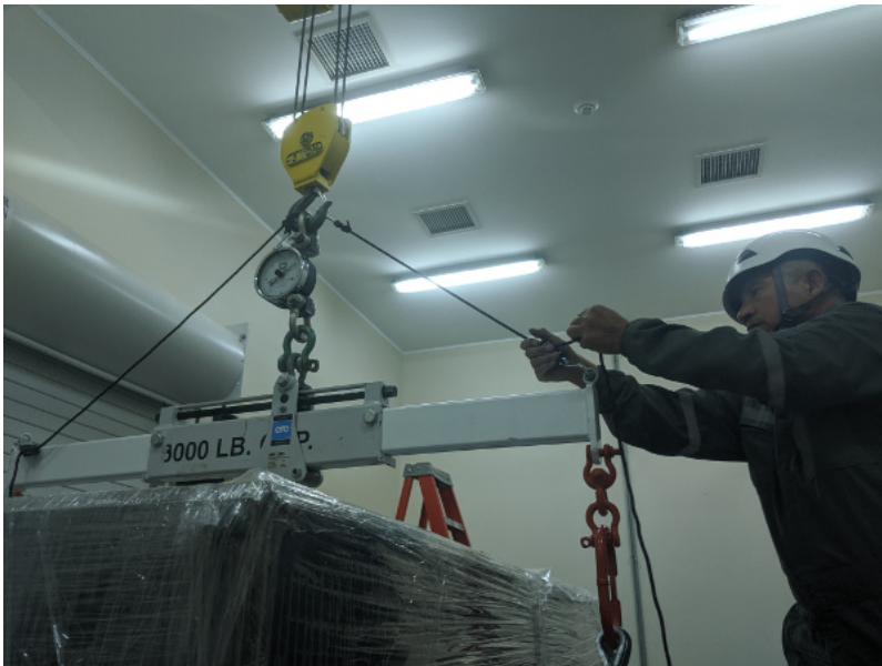
The triangle stabilizing ropes should be tight, but not become the lifting point for the load.
